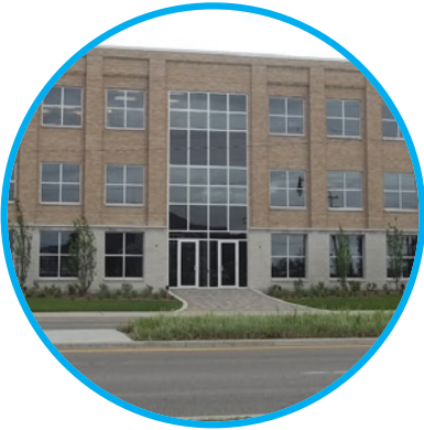
Office building framing the street with front yard landscaping
